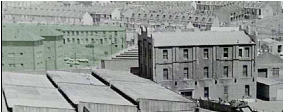
Figure 2.15 Looking westerly towards Mirrabooka in 1958 with the remnant terraces on Christie Street in the background
